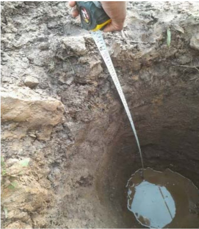
Excavated Fibre Pole hole
