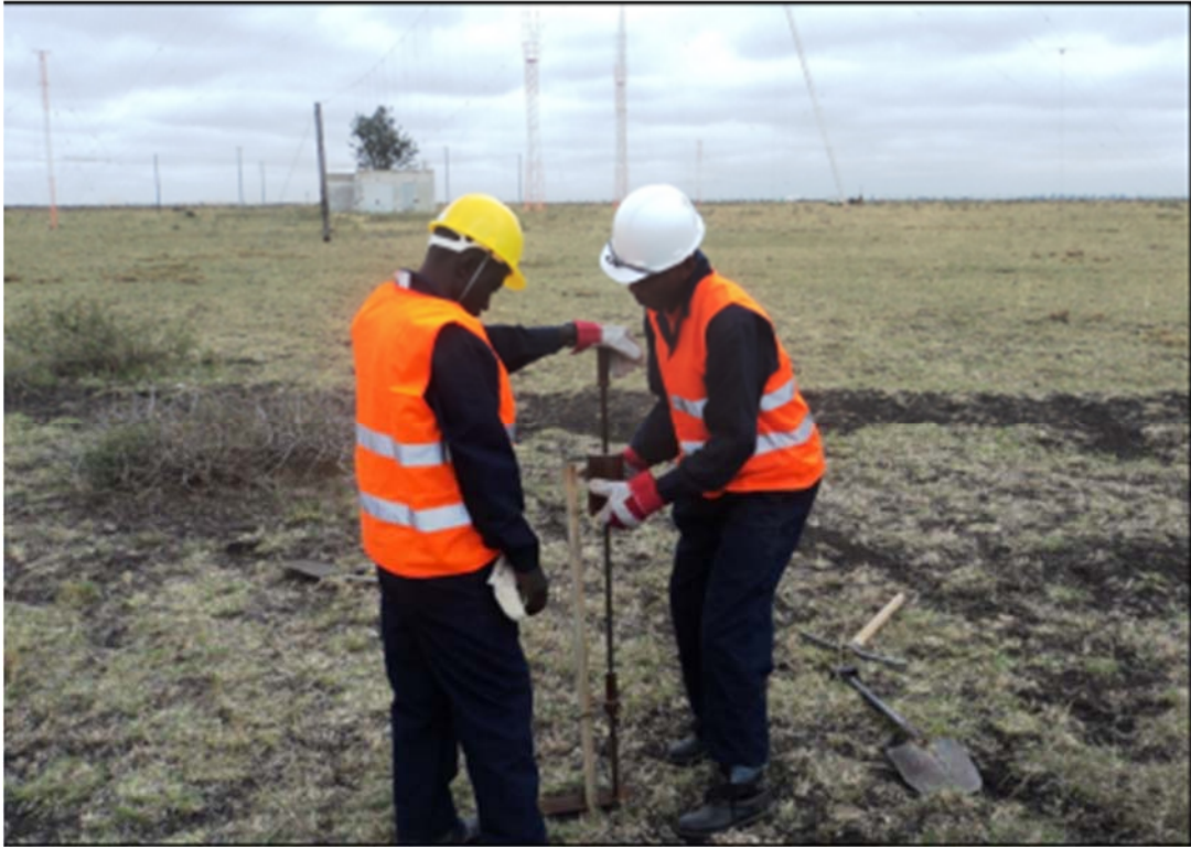
Photo showing DCP (Dynamic Cone Penetration) Test
