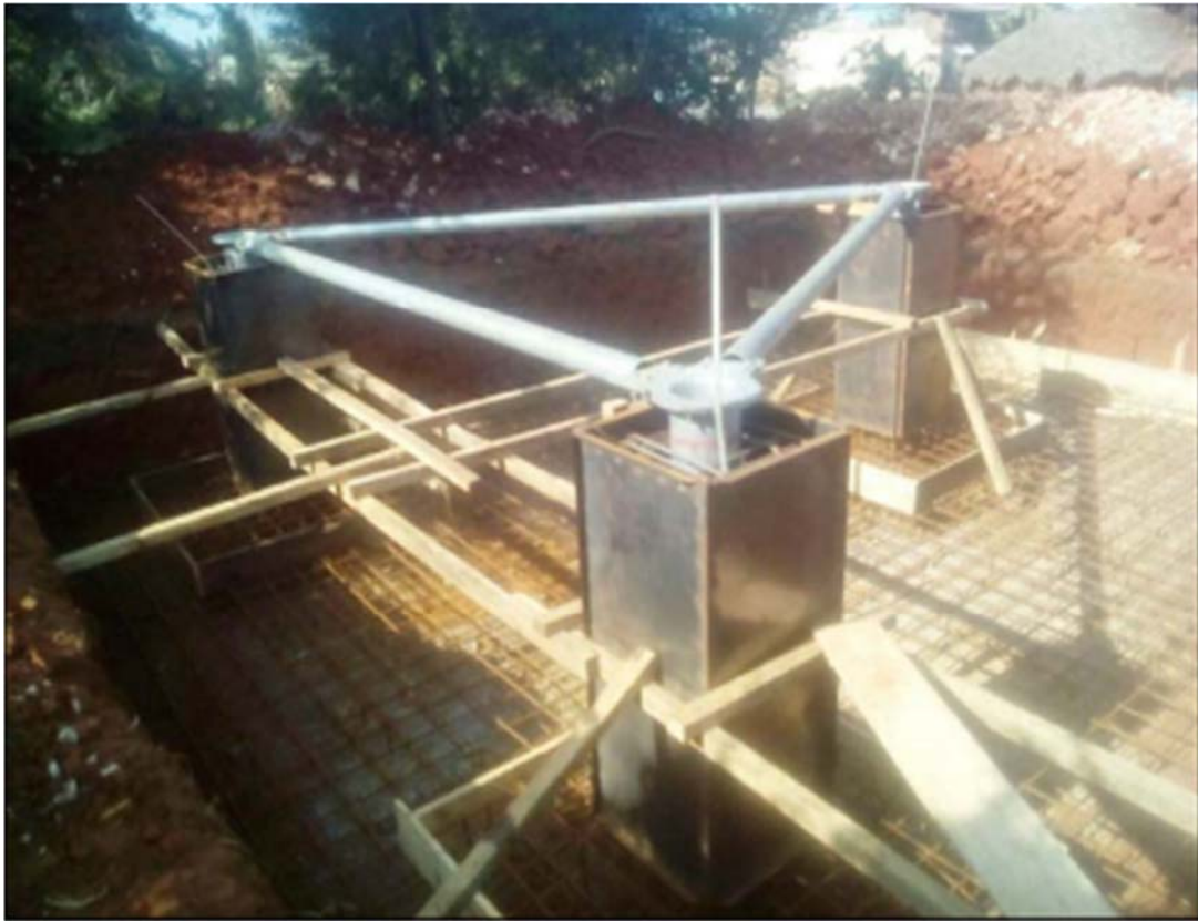
Formwork Ready for Casting
