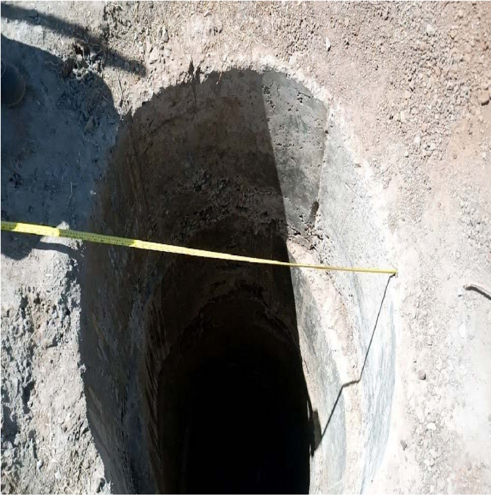
Tubestar monopole tower excavated foundation
