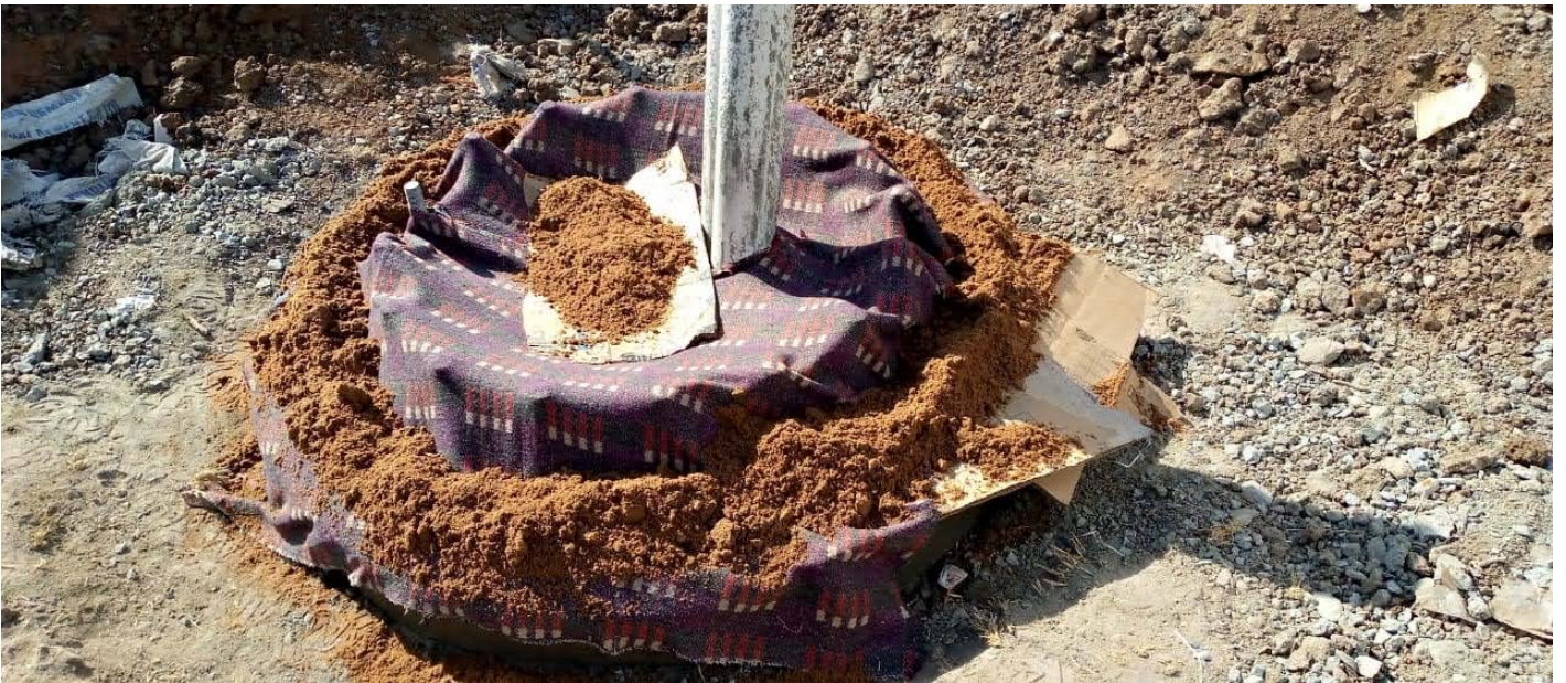
Monopole Tower foundation Curing
