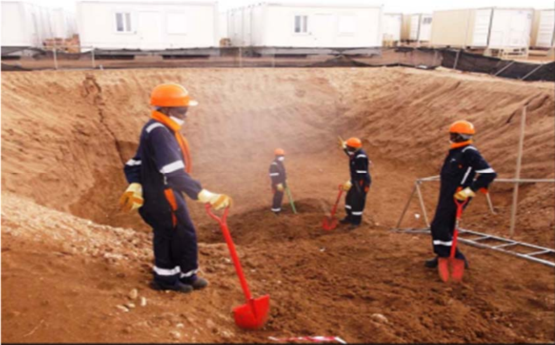
Site setting out and excavation for a raft foundation
