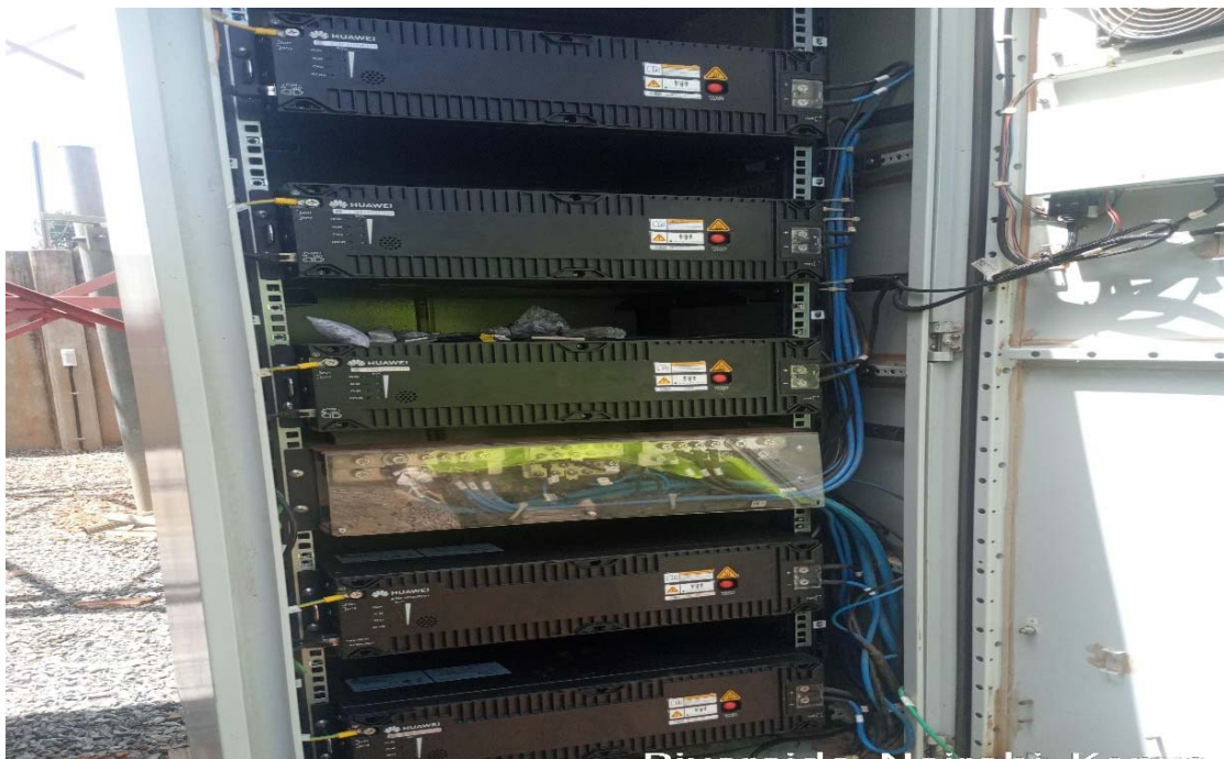
Solar Battery bank
