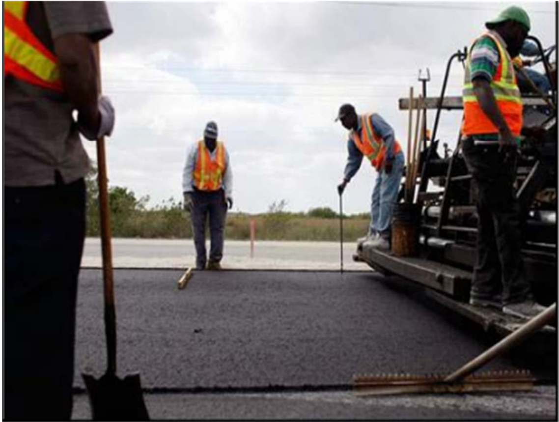
Compacting Asphaltic pre-mix
