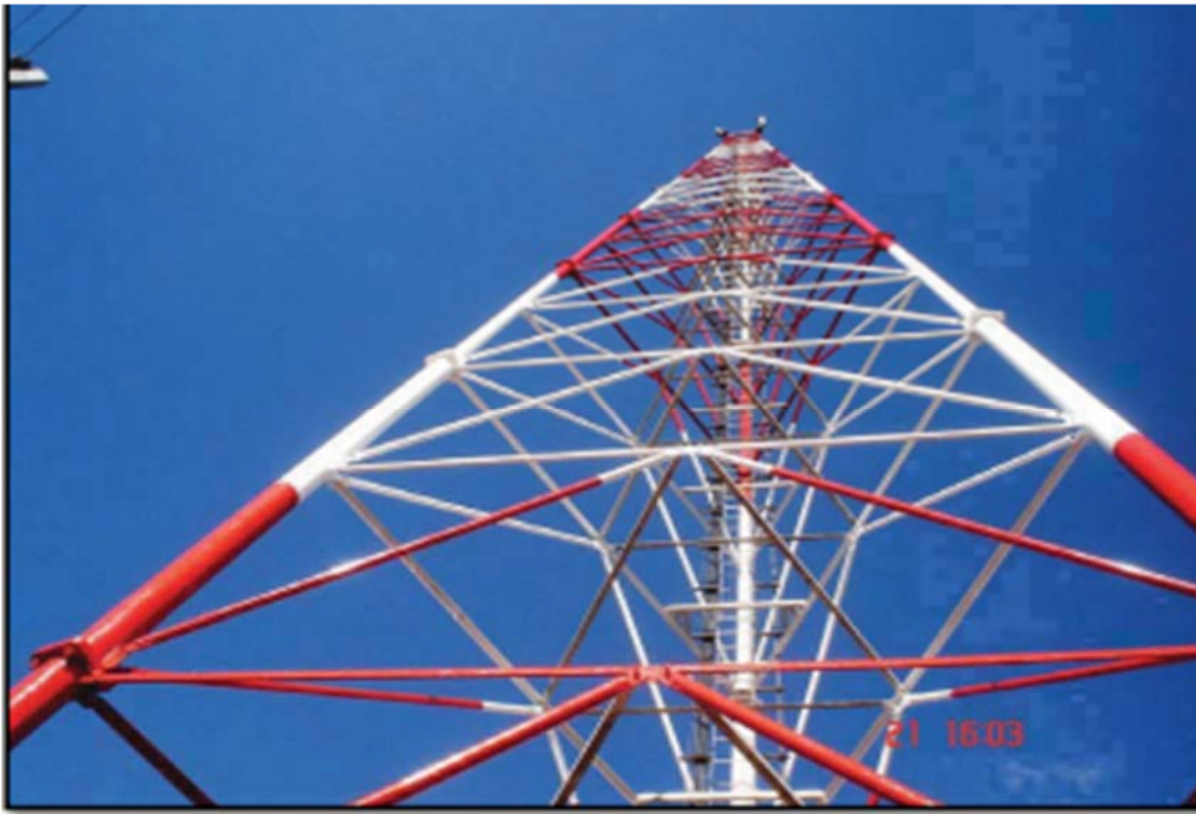
Top elevational view of tower
