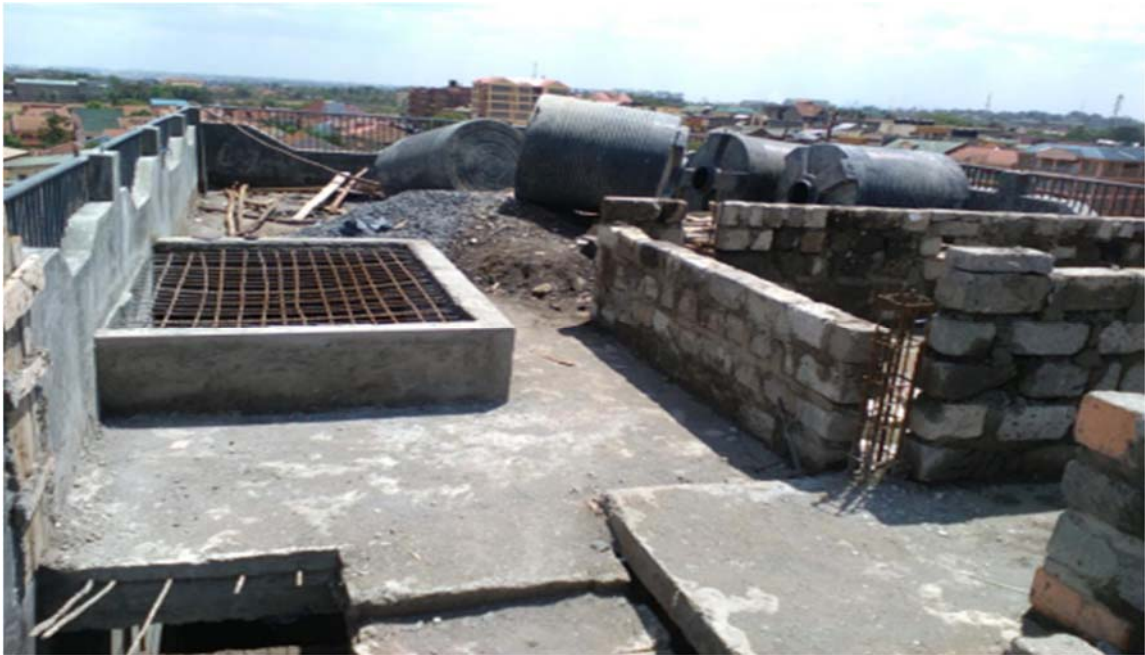
General view of the proposed site location on the GSM roof top (the area with water tanks)
