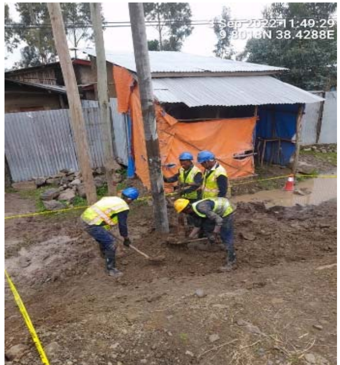
Backfilling/compaction
