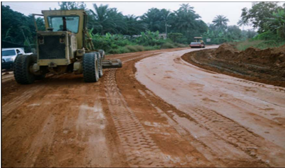
Grading compaction
