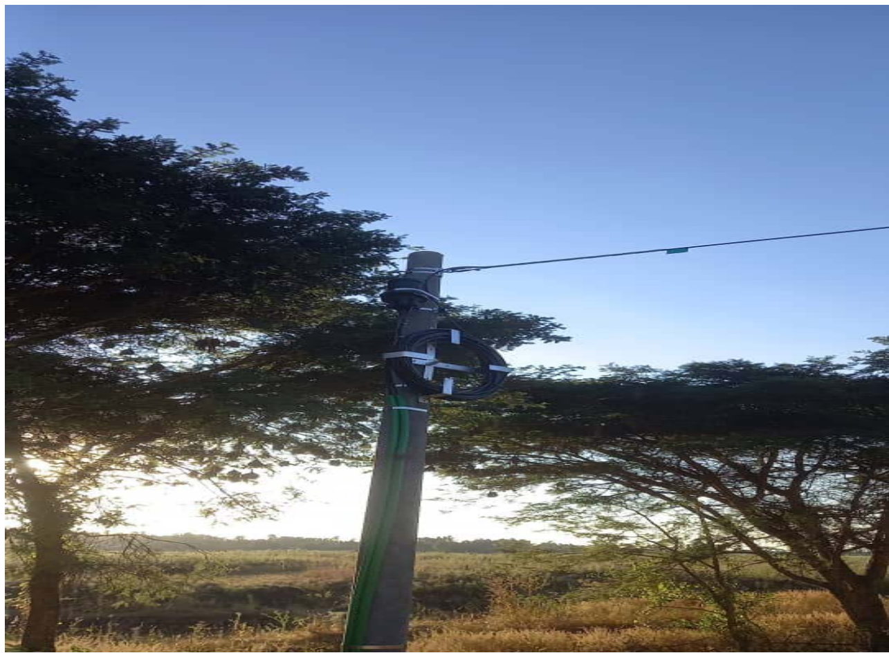
Fiber pole/cable installation
