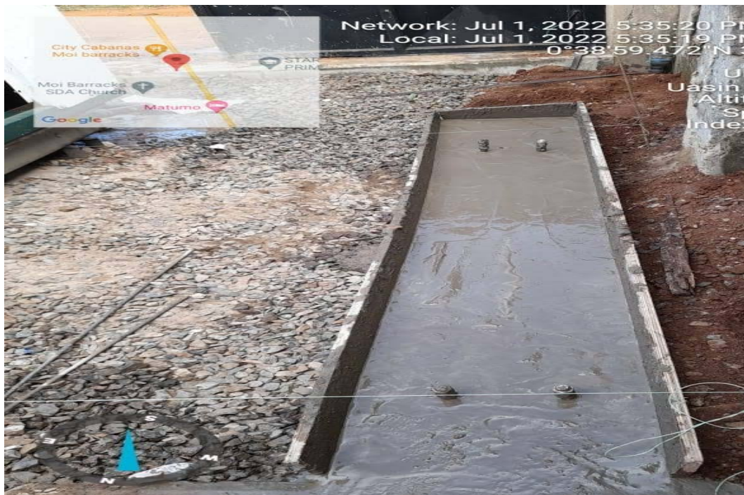
Reinforced concrete solar foundation beam casting done
