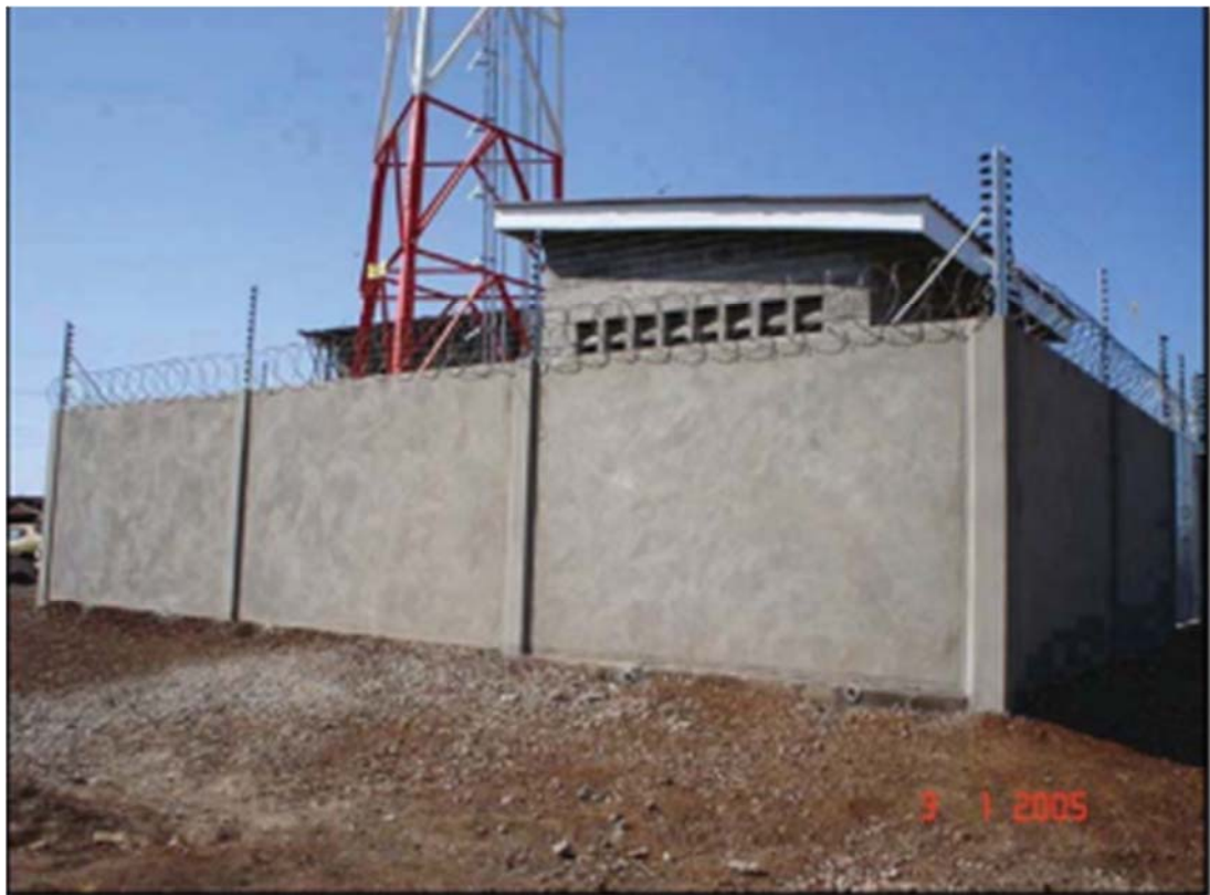
Site boundary wall with electric fence
