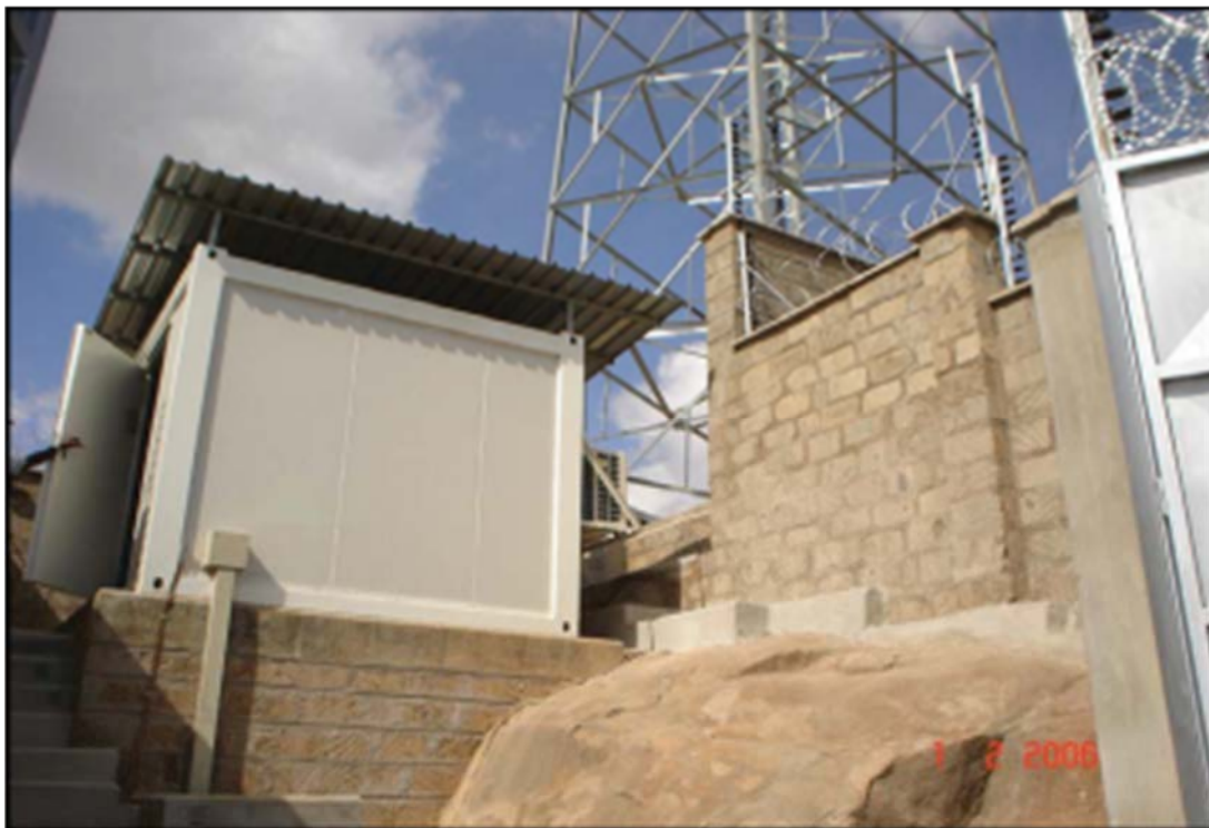
Indoor BTS location on a remote hill top site
