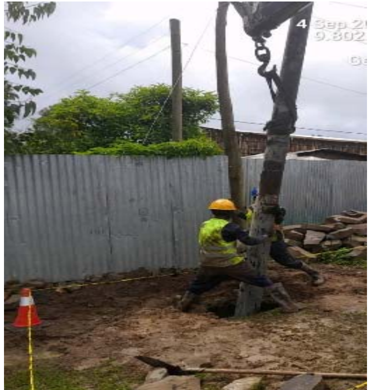
Fibre pole being erected
