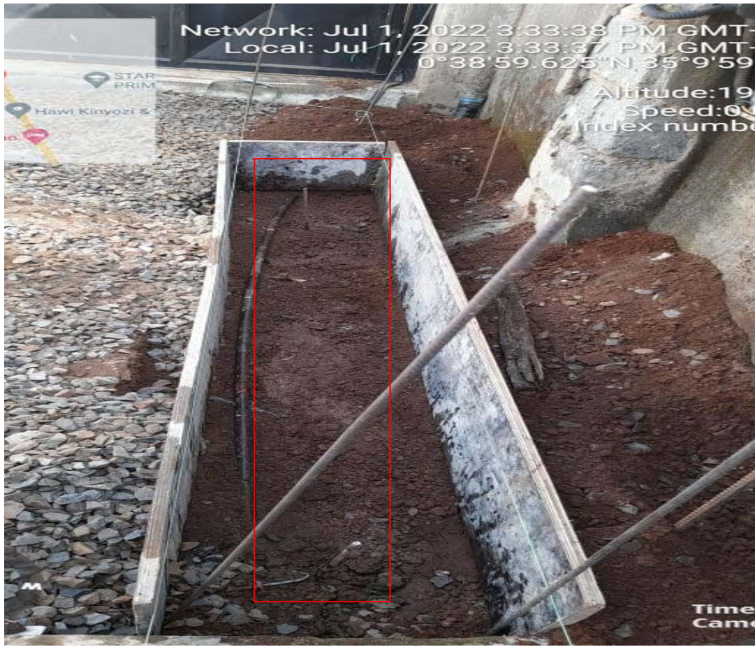
Formwork around excavated area for RC ground beam for solar structure
