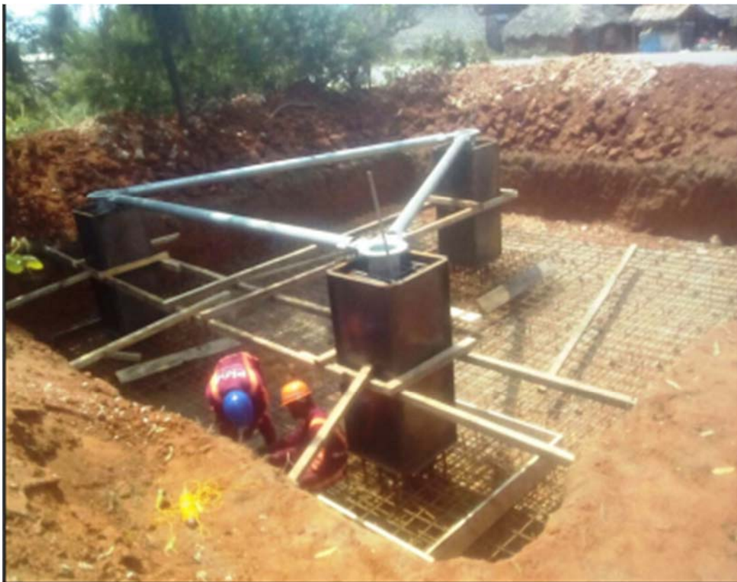
Tower Foundation Formwork Fixing
