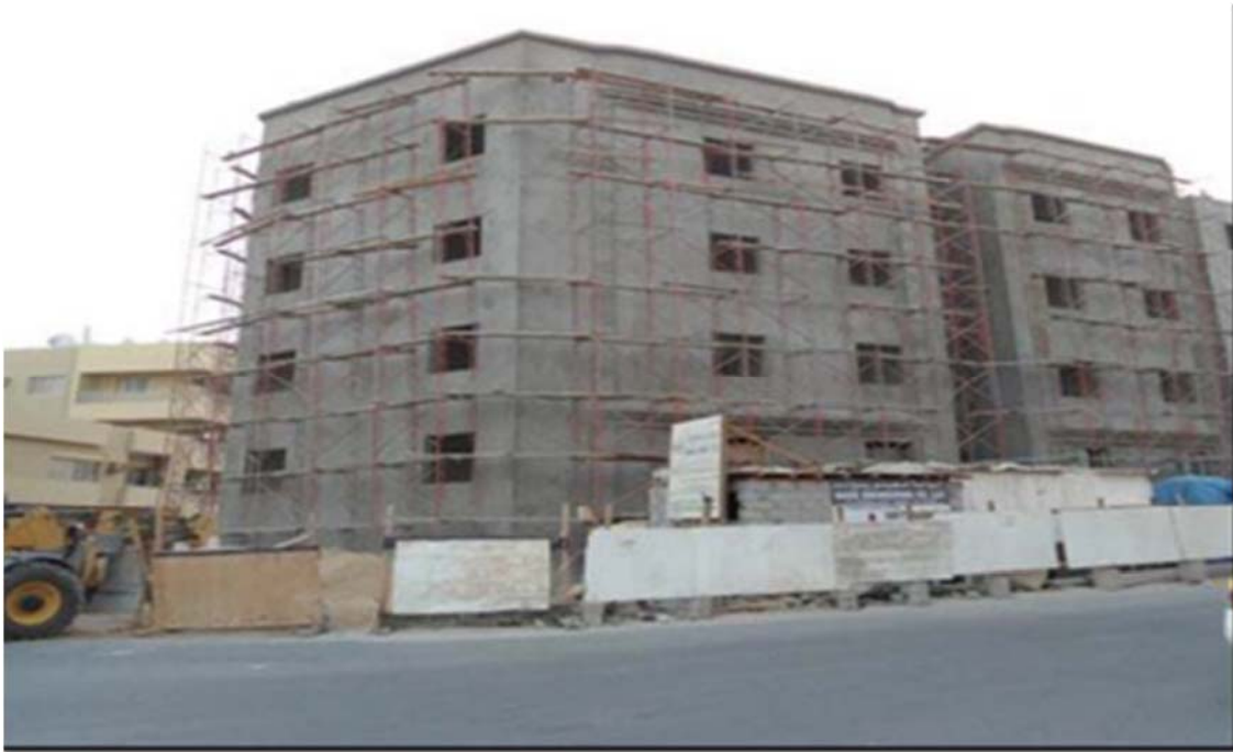
High – rise Apartments Construction
