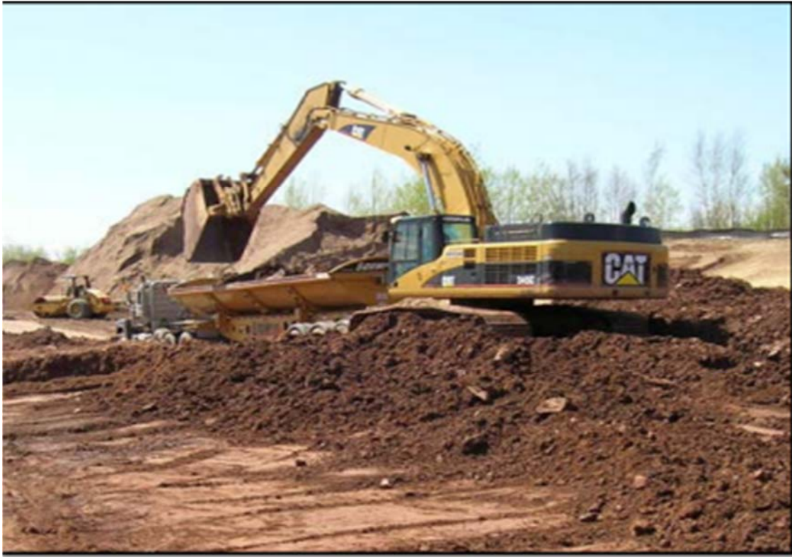
Road work construction
