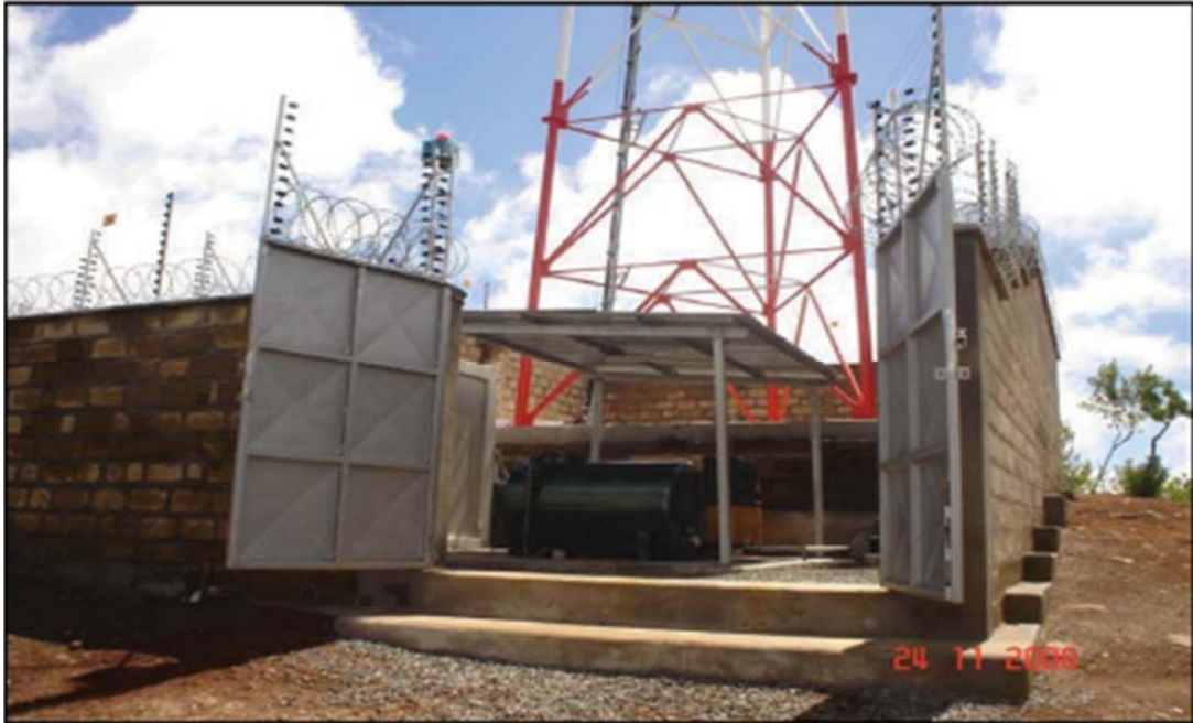
Site entrance view
