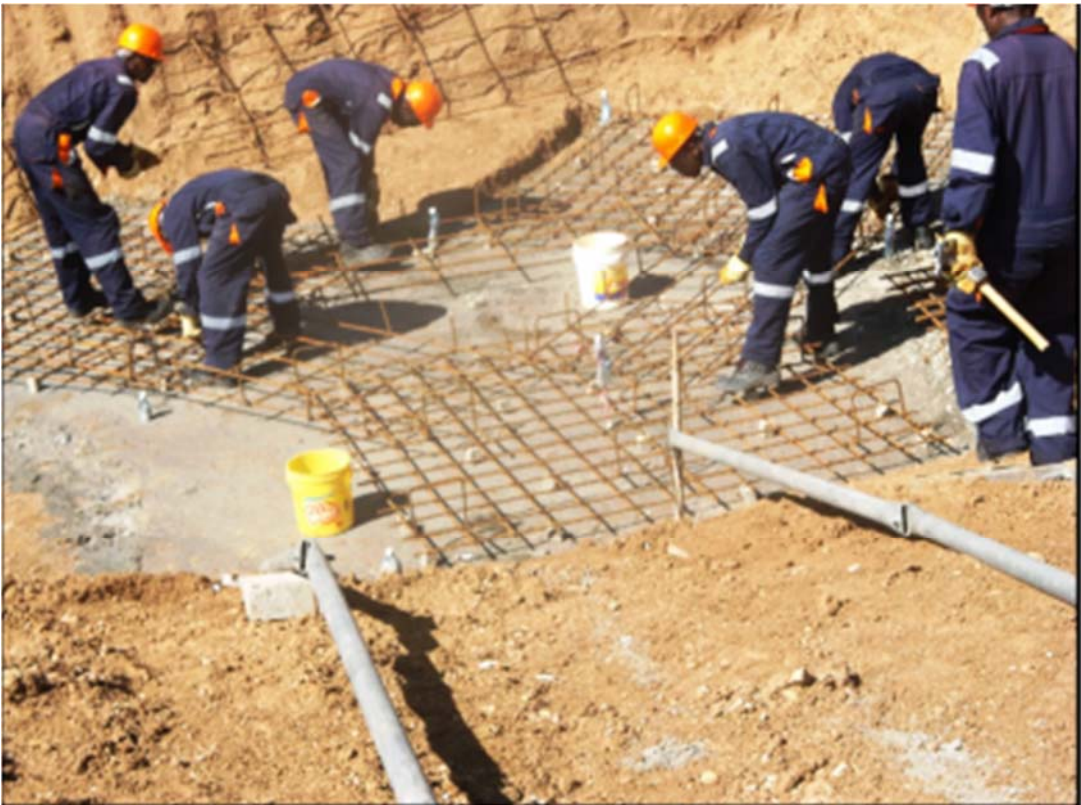
Tower Foundation Rebar arrangement and fixing
