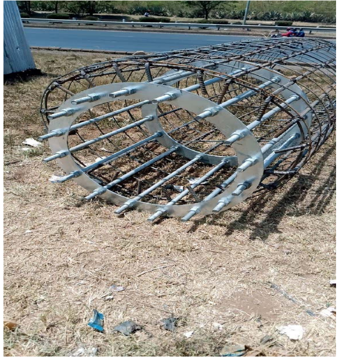
Tubestar rebar cage
