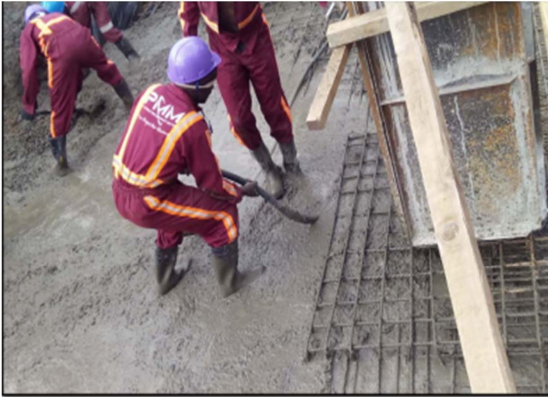
Tower foundation Casting ongoing
