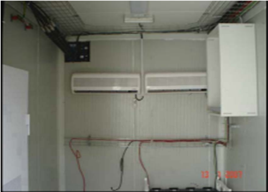
Jumper runs into Duamco of the BTS
