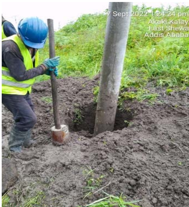
Fiber Pole erection/Filing
